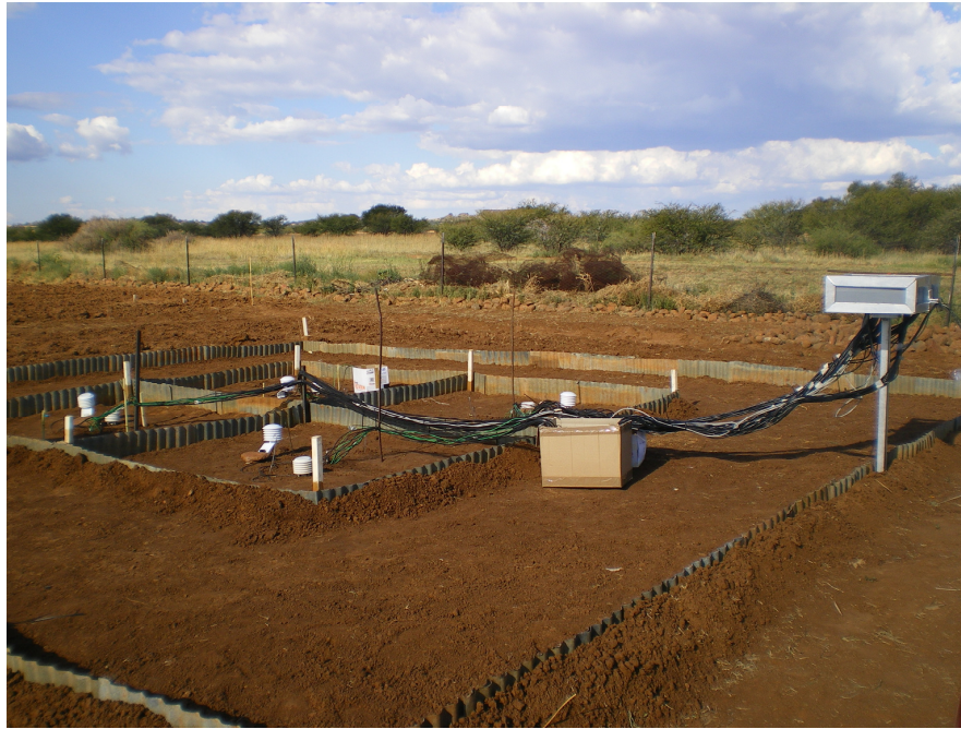
Figure A3.1 Photo showing ECH 2 O-TE and Vaisala probes cabling, CR1000 & multiplexer box and modem box holder
