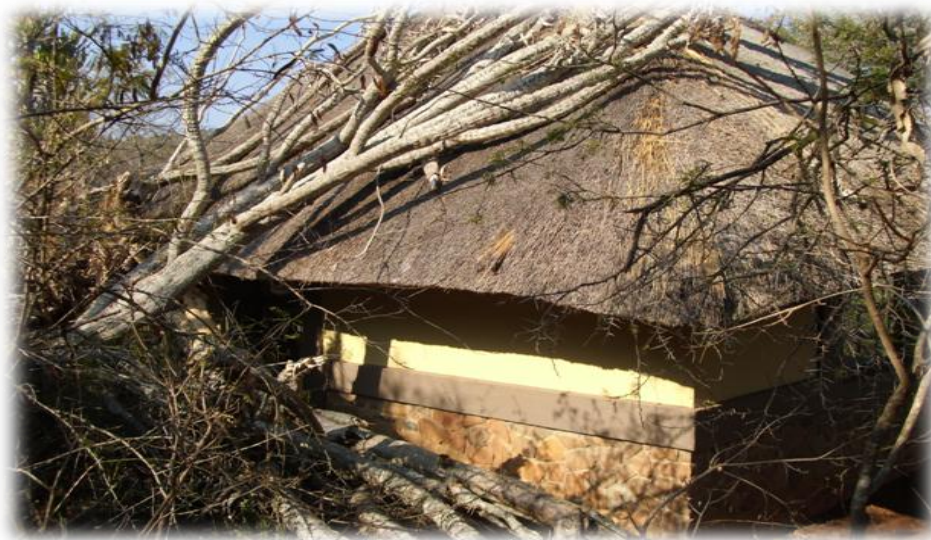
Plate 6.3: Deteriorating infrastructure in Ngome Community Game Reserve
