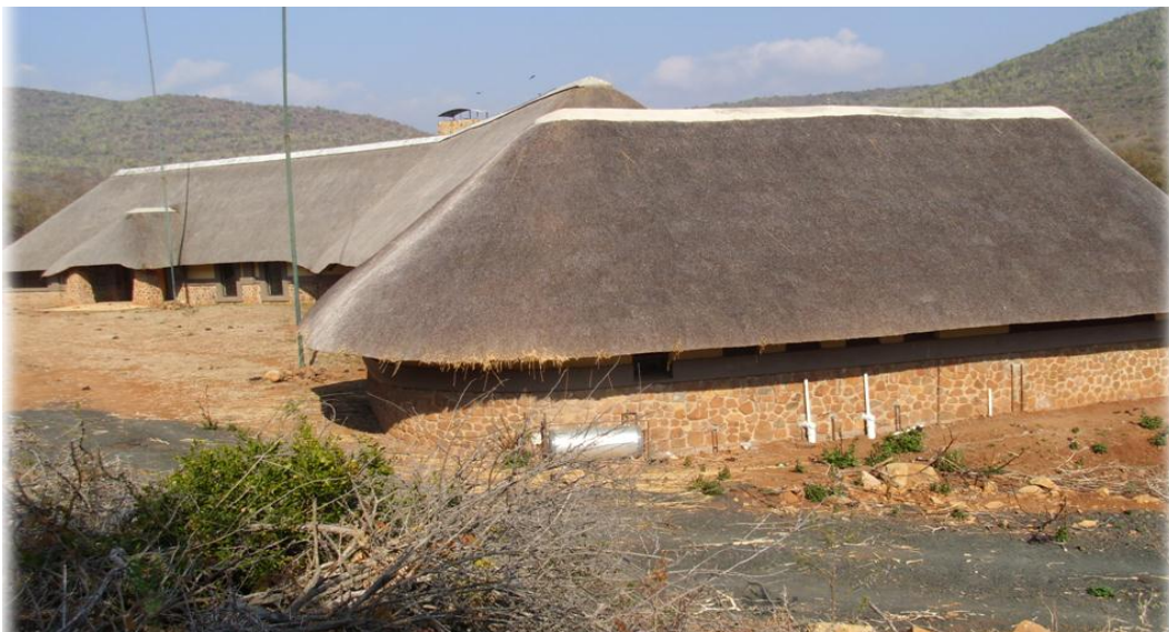
Plate 7.2: The newly constructed lodge and conference centre in Ngome Community Game Reserve
