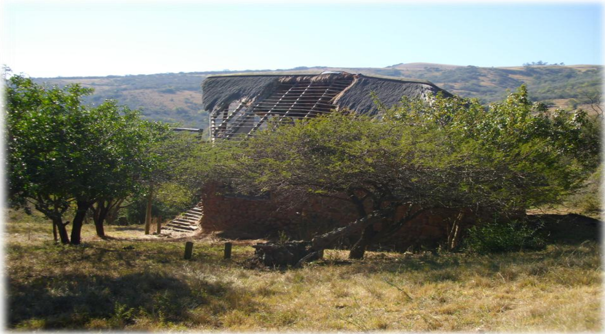
Plate 5.2: Vandalized lodge in what used to be Khobotho Game Reserve
