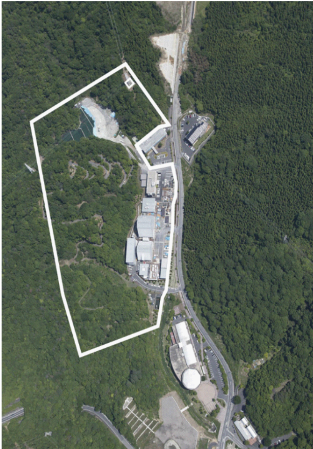
Fig. 3.14. Aerial view of the MIU site
