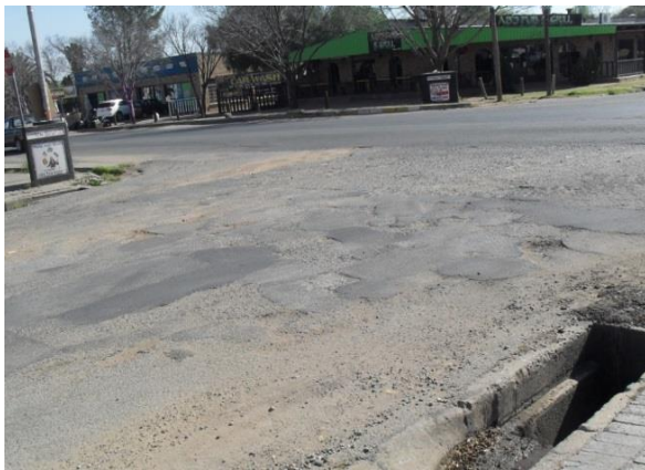
Figure 29: Lack of traffic signs at four way stop
