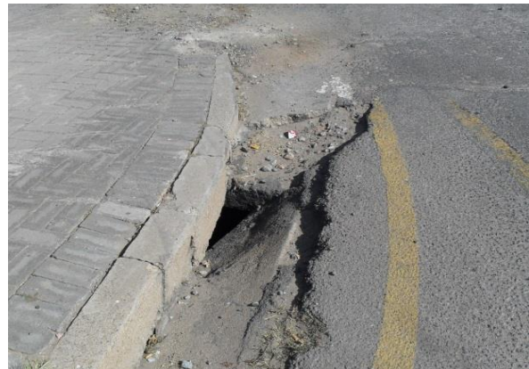
Figure 34: Current conditions of storm water drains in Parys (d)
