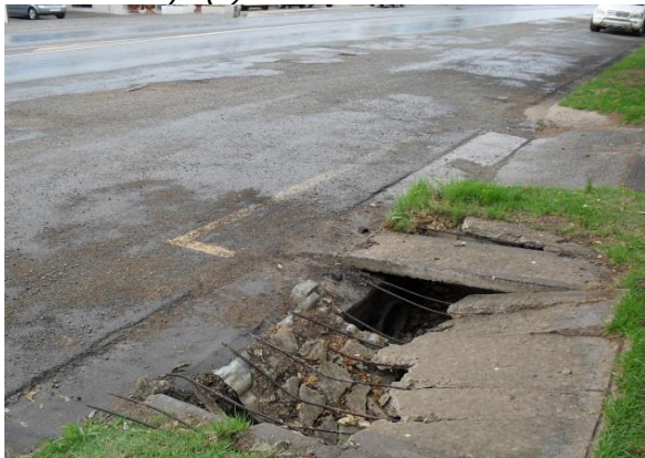
Figure 33: Current conditions of storm water drains in Parys (c)
