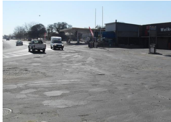
Figure 28: Lack of traffic signs at major entry road (R59)
