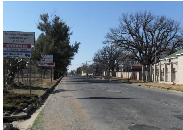
Figure 17: The condition of the R53 entering Parys
