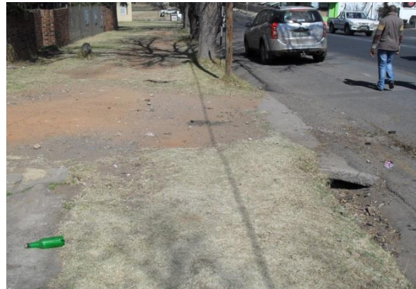
Figure 21: Current conditions of sidewalks in Parys (b)
