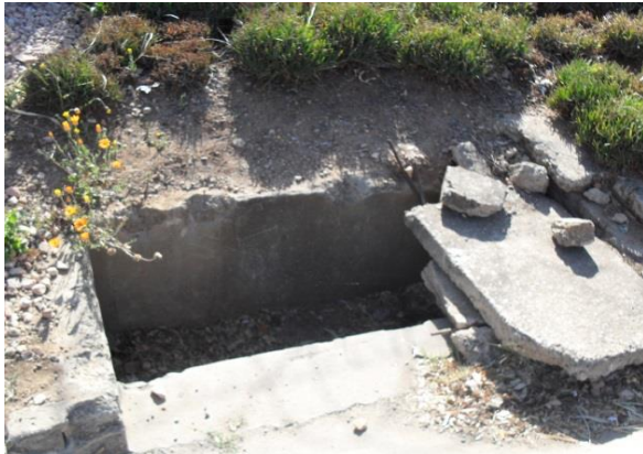
Figure 31: Current conditions of storm water drains in Parys (a)
