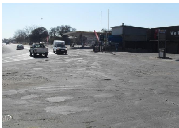
Figure 15: The condition of the R59 entering Parys via Loop Street
