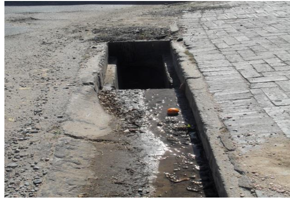
Figure 32: Current conditions of storm water drains in Parys (b)
