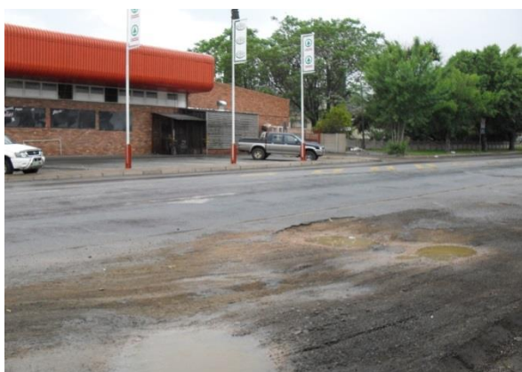
Figure 14: The condition of the road in Breë Street
