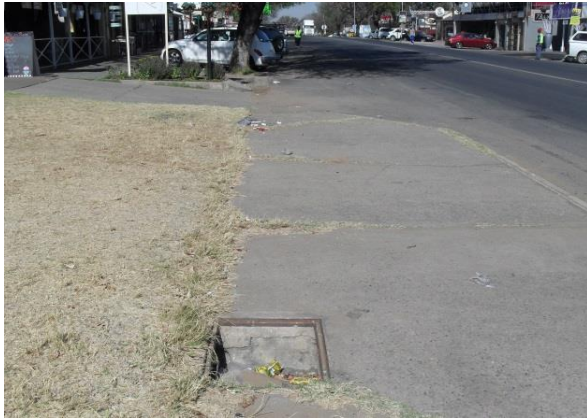
Figure 35: Current conditions of the general appearance of Parys (a)
