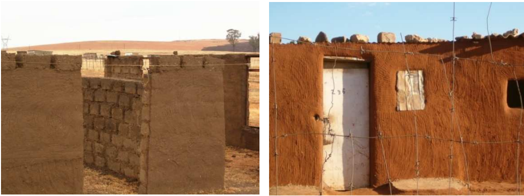
Figure 6.2 Adobe (traditional un-stabilised sun-dried mud bricks) in Botshabelo
