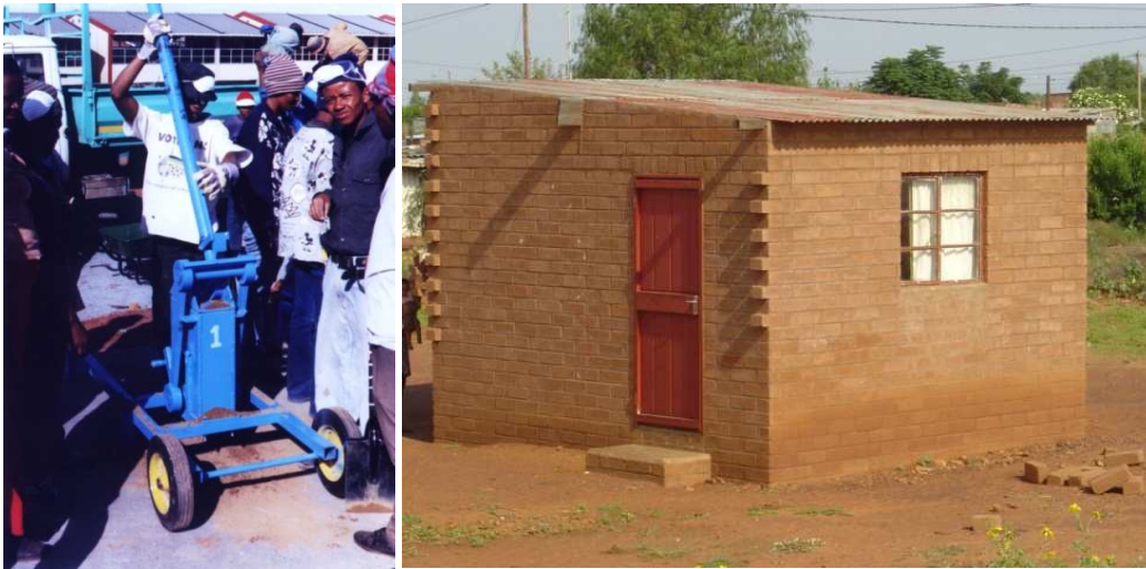
Figure 8.3 Use of cement stabilised compressed earth blocks (CEB) bought from local entrepreneurs for a self-help house in Bankhara Bodulong, near Kuruman
