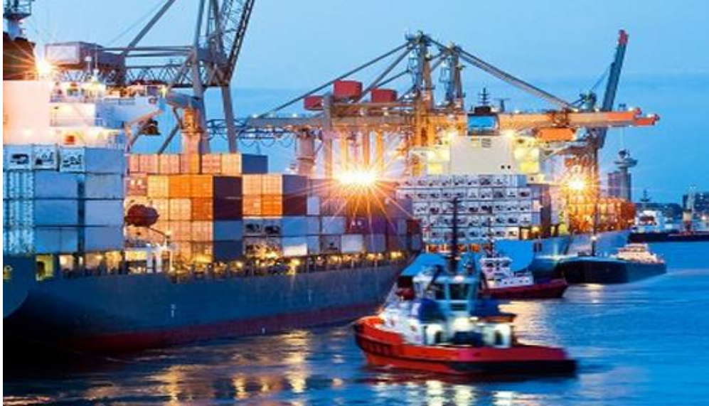
Figure 4: Kenya's new terminal at Mombasa port in 2016
