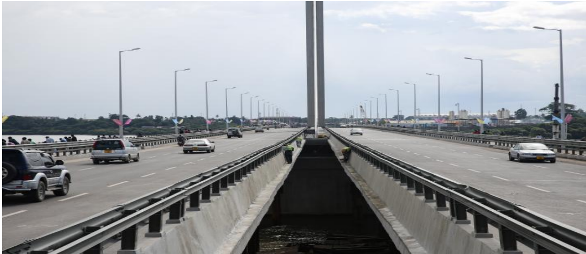
Figure 6: The completed 32 metre wide Kigamboni Bridge
