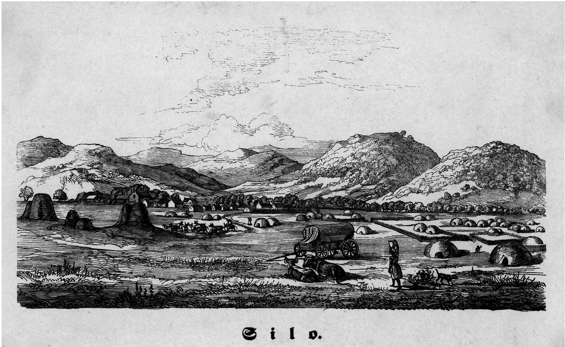
Silo (with the church in the background left). 1
