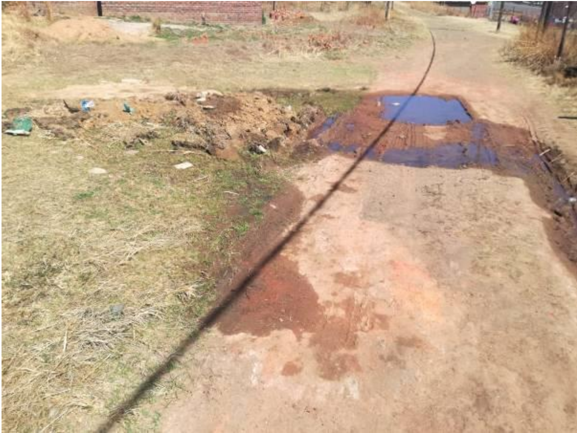
Figure 5.22: Water leakage from a MAP Water pipeline in the Bolata village on 7 February 2019
