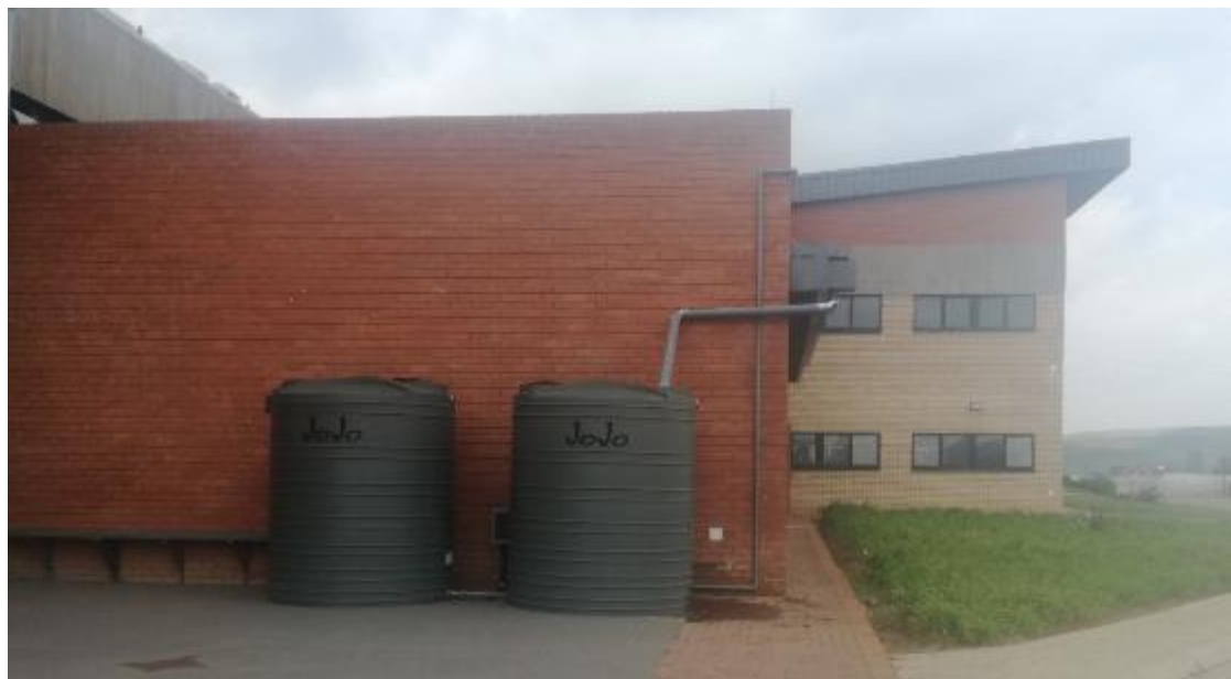
Figure 7.10: Water harvesting of rainwater from the University of the Free State, QwaQwa Campus on 7 February 2019
