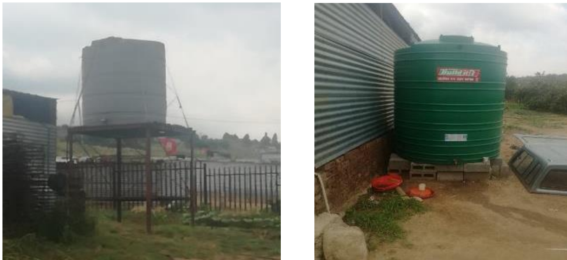
Figure 7.11: Mocwagae Poultry's 10 000 ℓ (left) and 2 500 ℓ (right) water tanks 7 February 2019
