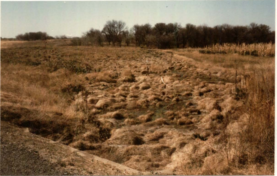
Fig. 2.6 Site no. 8: A marsh formed by seepage from a dam.
