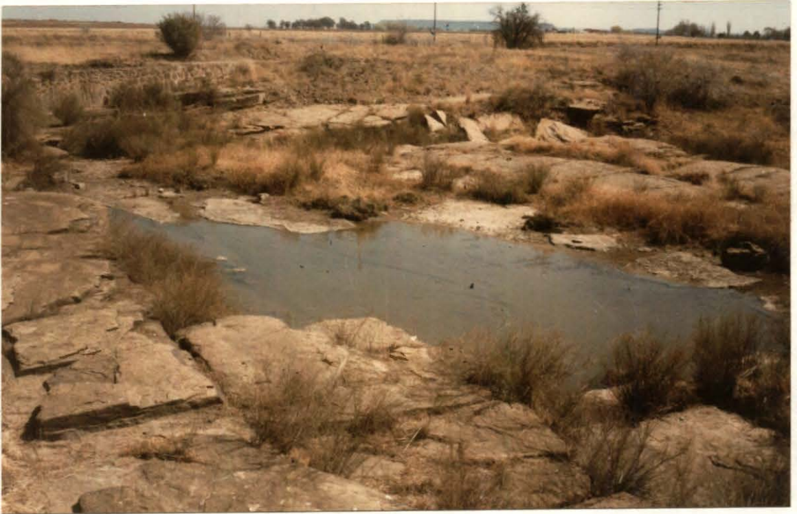
Fig. 2.2 Site no. 1. Shallow rock seepage pools situated below a stone and concrete weir.
