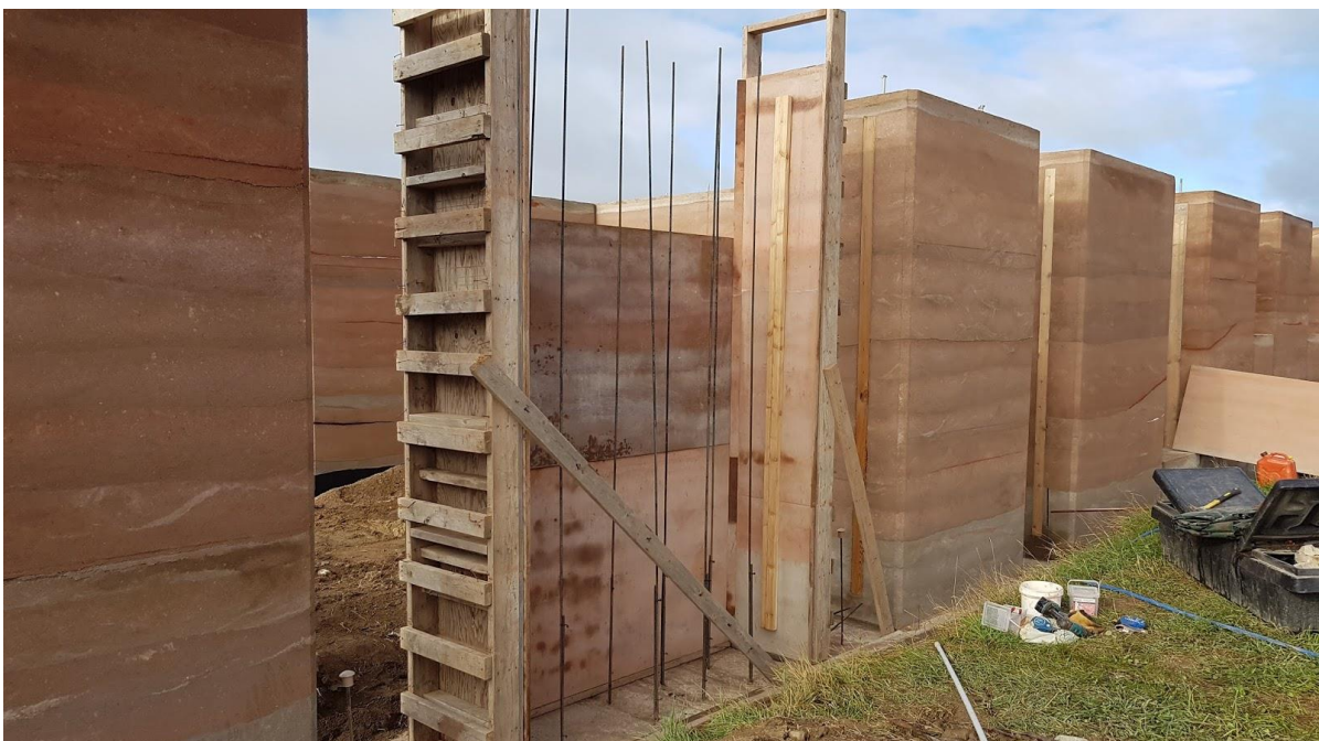
Fig 47. Rammed Earth Walls (PKBN, 2016: online)
