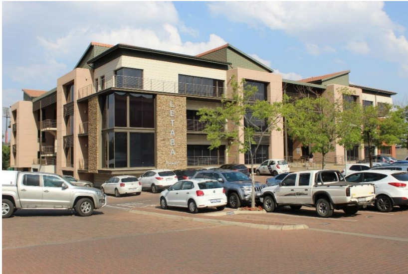
Pictures 10: NDMC rented offices (3rd floor)
