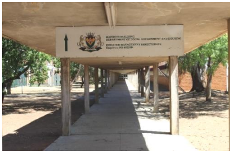
Entrance from main gate 1
