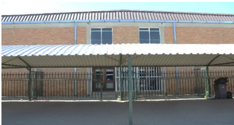
Entrance into building
