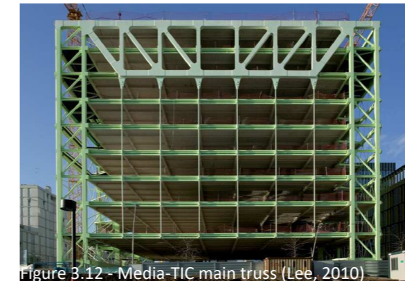
Figure 3.12 - Media-TIC main truss (Lee, 2010)
