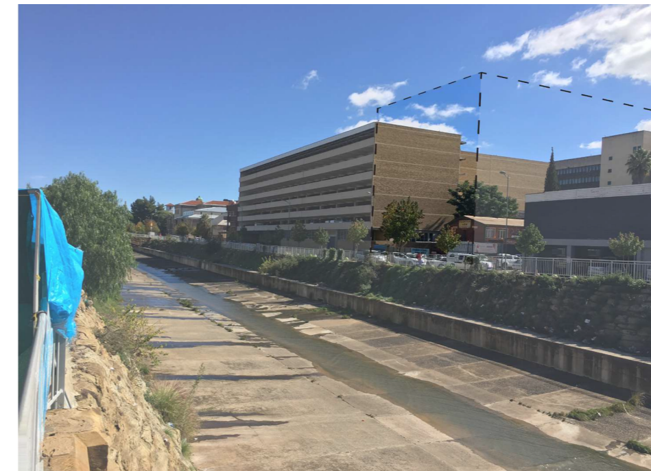
Figure 2.4 - Canalization of the spruit
