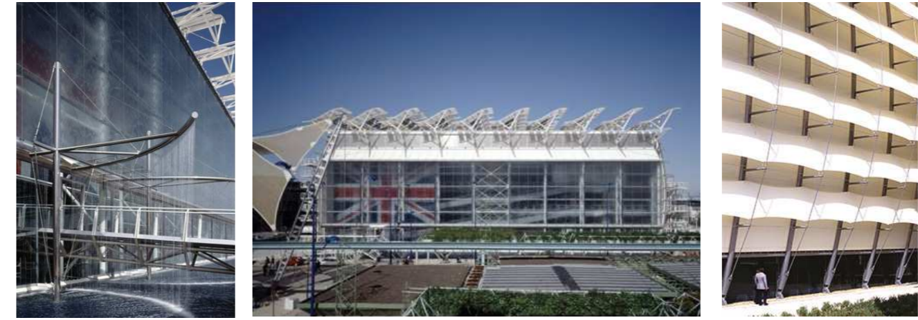
Figure 2.42-44 - 1992 British Pavilion climate control systems (Grimshaw Architects, 2019)
