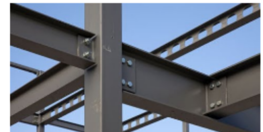
Fig.73 - Connections used in steel column and beam construction. Source: online
