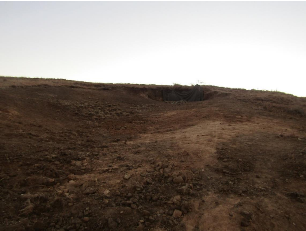
Fig. S5.1b: Flattening of the site, with displacement of soils around the initial eroded site, taken during July 2018.
