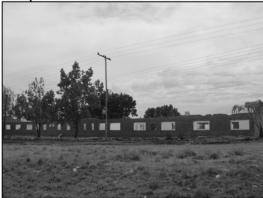
Photograph 9 Dilapidation of Poloko Sanatorium, 2003
