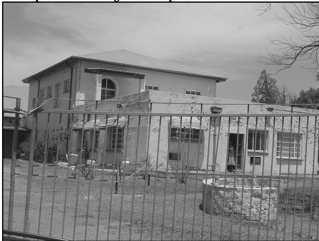
Photograph 7 Dilapidation of Allanridge Chest Hospital, 2003
