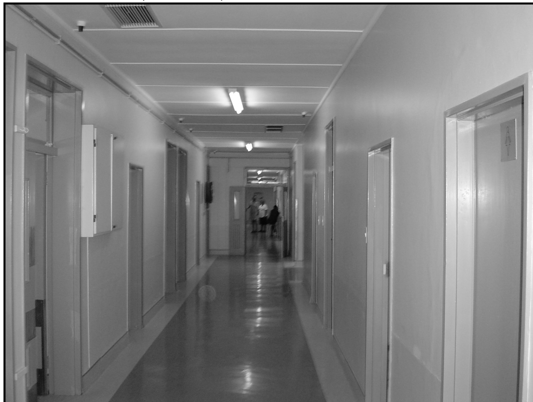
Photograph 16 Extraction fans, MDR-unit, 2003
