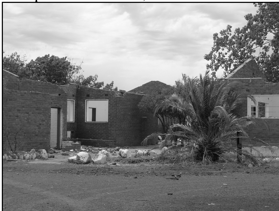
Photograph 9a Dilapidation of Poloko Sanatorium, 2003
