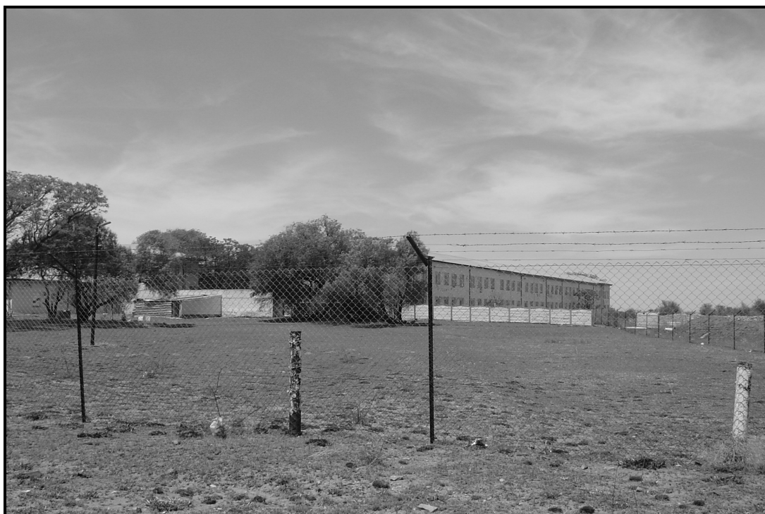
Photograph 8 Infrastructure of Allanridge Chest Hospital, 2003
