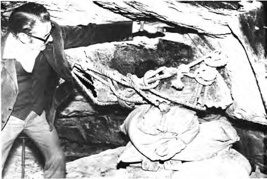
Mr Hannes Els, foreman of Roberts Construction, Welkom, explains how the drilling into the rock face was undertaken to ensure the safe removal of the painting.
