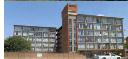
THE CONCRETE-FRAME APARTMENT BLOCK
