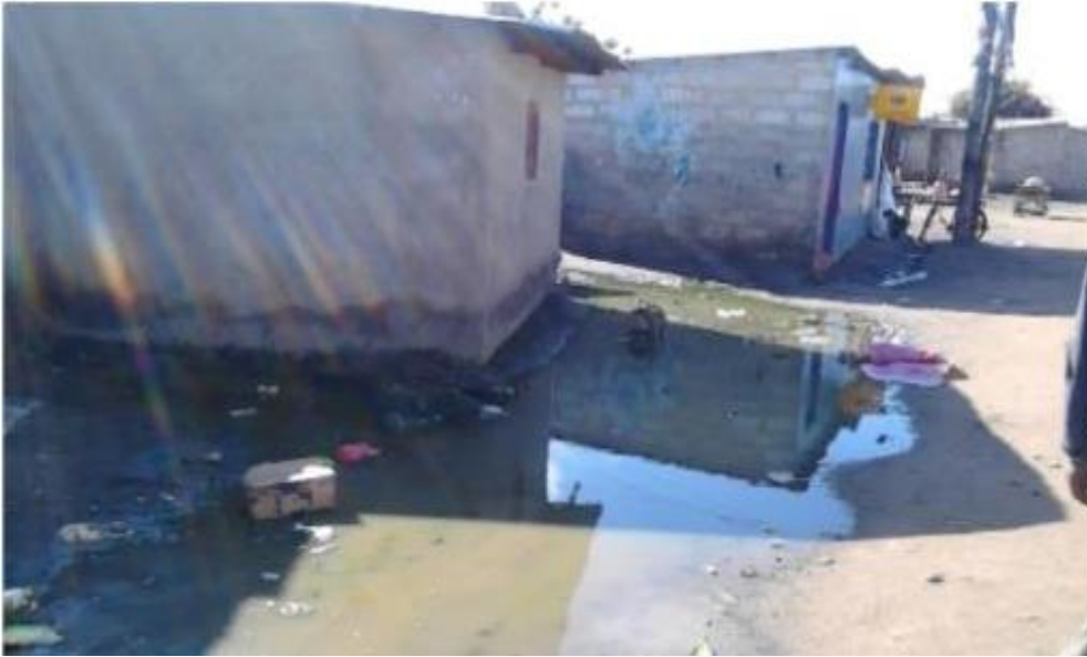
Figure 4.3 Physical environment in Misisi Compound
