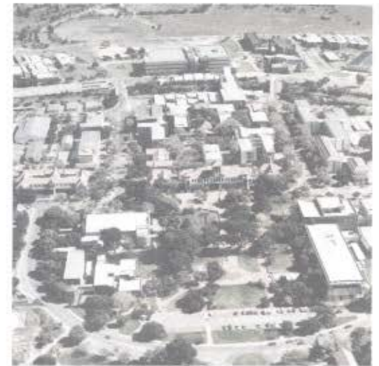
Fig: 2004: Areal view of campus with Thakaneng Bridge
