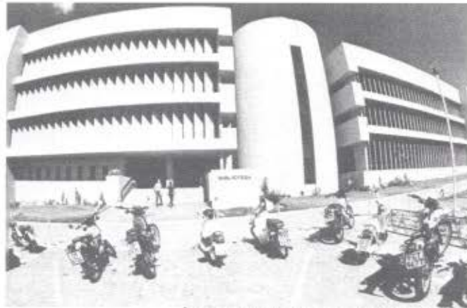
Fig: 1984: West facade of new Sasol Library
