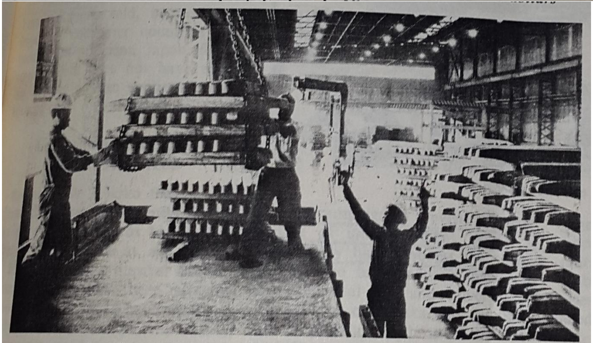
Figure 5.2: Top picture shows Nkana's new Roast Leach Electro-win Cobalt Plant in June 1984, with a capacity of 2,400 metric tons of cobalt metal per year. The bottom photograph shows workers loading copper bars at Nkana Division. Source: Both pictures taken from The Courier , No. 85 (1984), 20-1.
