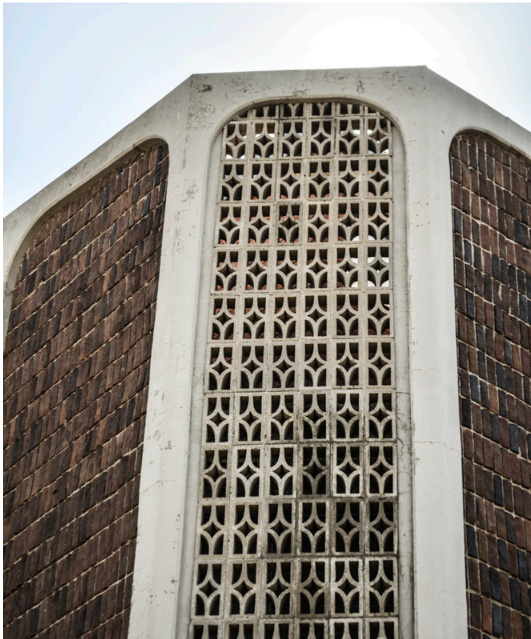
Concrete air bricks
