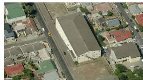
WESTERN AERIAL PHOTOGRAPH
