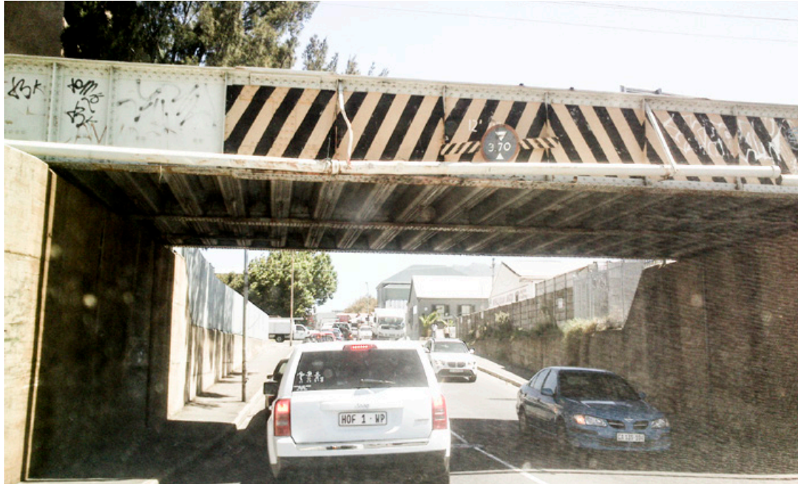
Bridge over Rockley Road
