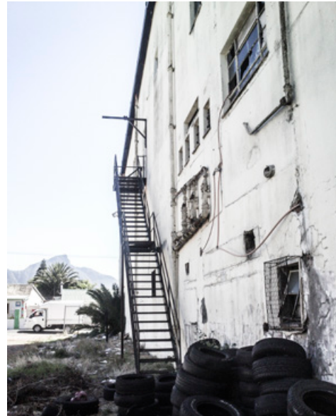
Fire escape and broken windows
