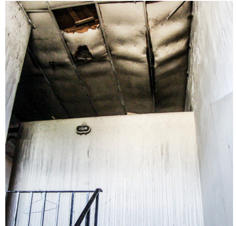
The circulation shaft that also got damaged by the fire
