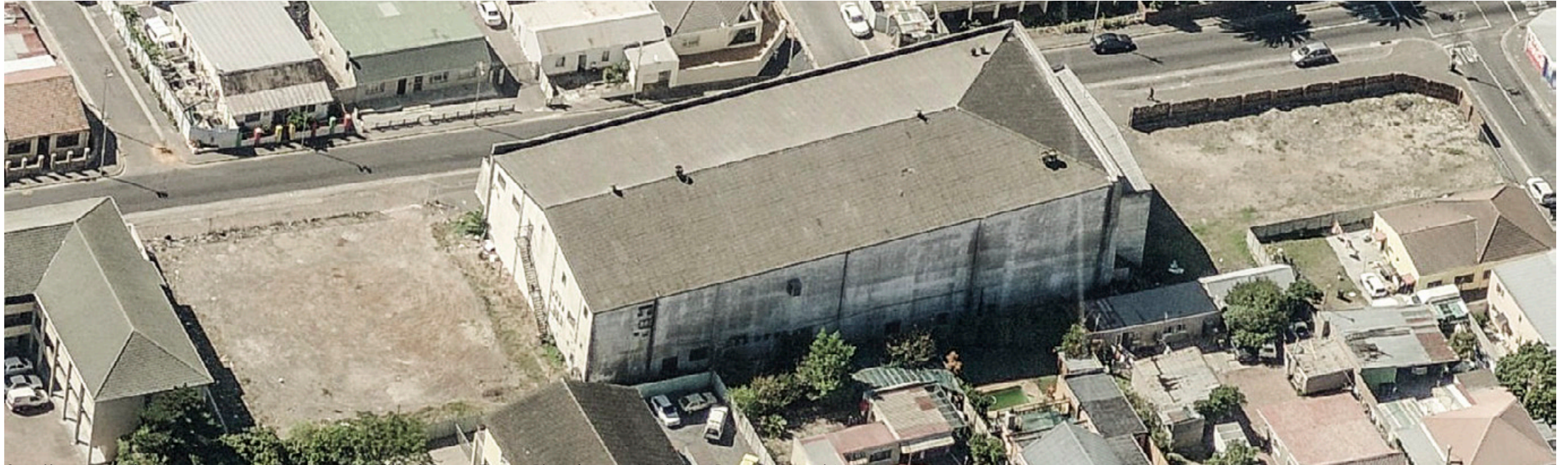
Southern aerial photo Obtained from: City of Cape Town, Planning and Building Development Management (2014)
