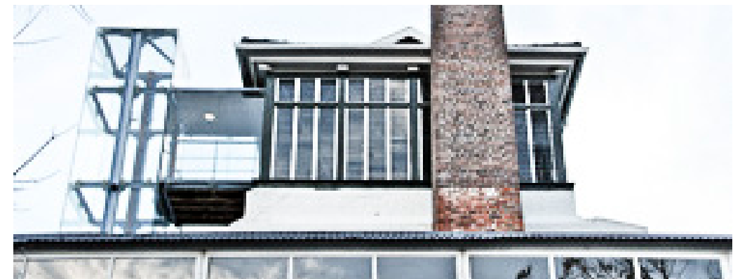
Brick chimney with its counterpart, glass elevator Online image. Available at: http://www.artefacts.co.za/imgcat/thumbnails/SABVisCnt62.jpg
