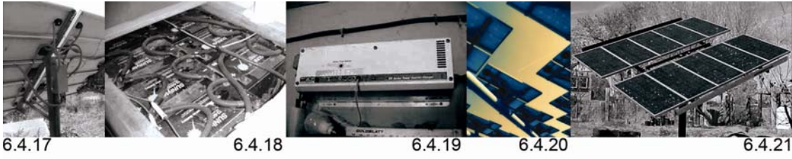
6.4.17. Cables at the back of the sunpanels. 6.4.18. Gel type batteries for storing electricity . 6.4.19. An inverter that inverts power from direct to alternating current. 6.4.20.- 6.4.21. Solar panels mounted on steel structures (Solar panels are black to absorb solar energy and transforms it into electrical energy. Therefore a minimum amount of heat is reflected towards the surrounding structure. This makes solar panels ideal for the sunroof)
