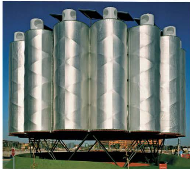
Illustration 4.37 Air Tree Pavilion. The outer skin is made from high-density, multilayer polyethylene films and aluminium. [Emilio P Doiztua,2009:Online]
