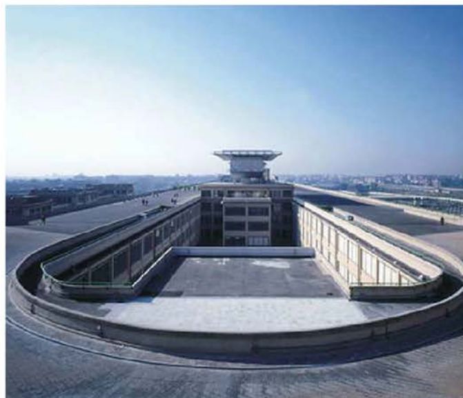
Illustration 4.19 Old Rooftop Test Track. [RPBW, n.d.:Online]
