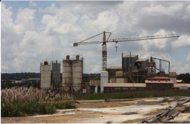
Crown Mines Reclamation Plant, Main Reef Road West.
