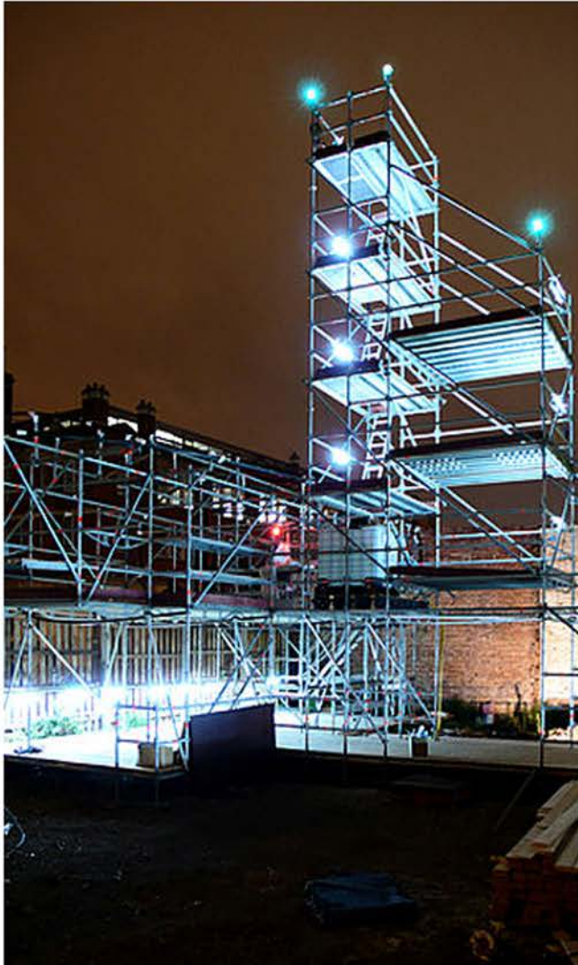
Illustration 4.30 Temporary Steel Structure. [Agnese Sanvito, 18 Julie 2008: Online]
