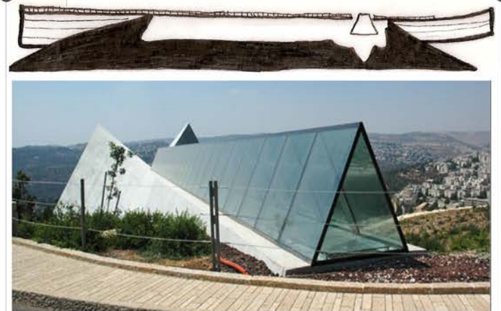
Illustration 4.25 The structure penetrates the mountain from one side to the other, with both ends dramatically cantilevering into the open air. [Yad Vashem, n.d.:Online]
