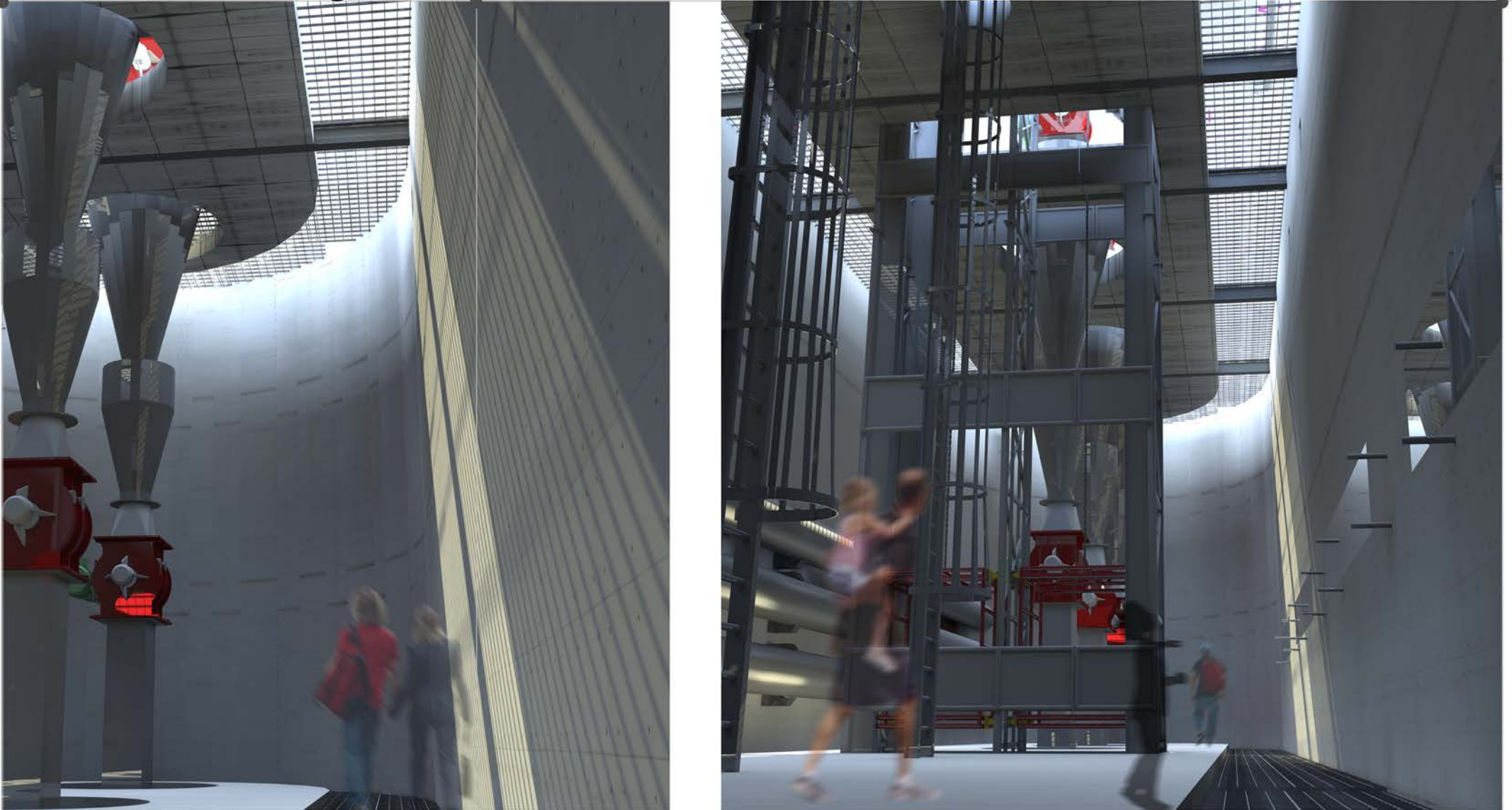
Illustration 6.48. Deep water pumps in existing mine shafts.
