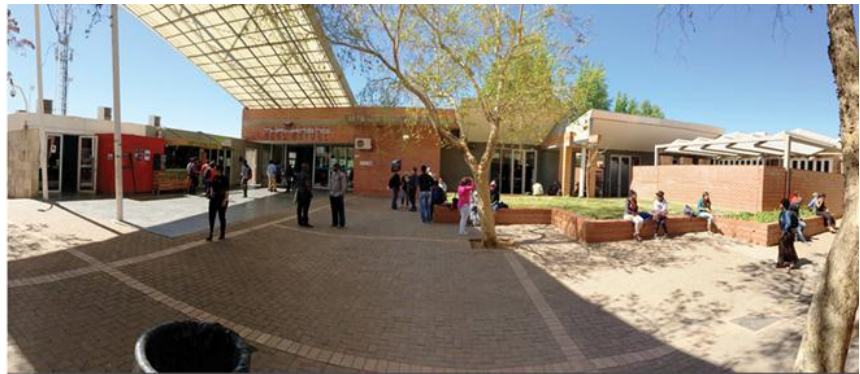
b Open forecourt of the Thakaneng Bridge with comfortable spaces for socialising.
