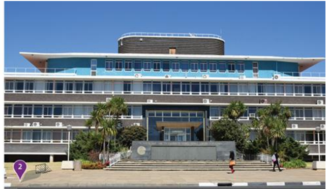
2 b Buildings of high architectural value.
